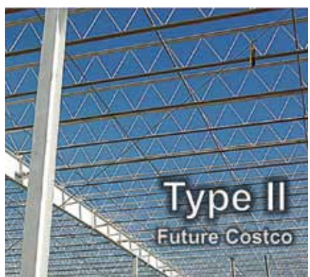
Type II building featuring unprotected steel.
