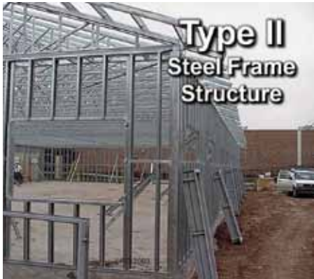
Lightweight steel frame structure (paint it brown and it would look like wood).
