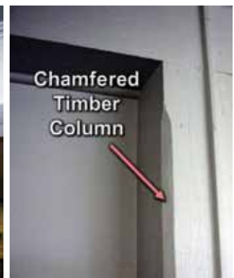
Heavy-timber edge chamfer.
