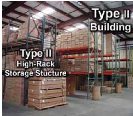
Type II high-rack structure within a Type II building.
